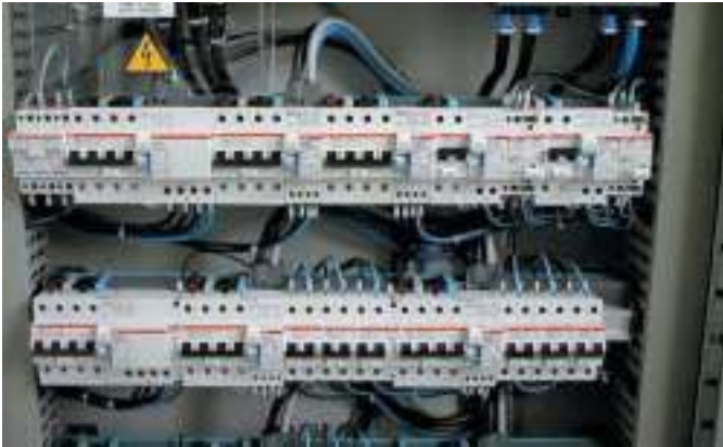
Due different single-phase circuits on a single 24 module DIN rail
